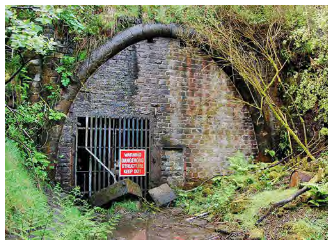
The north portal of Queensbury Tunnel. Photo Phil Davison
